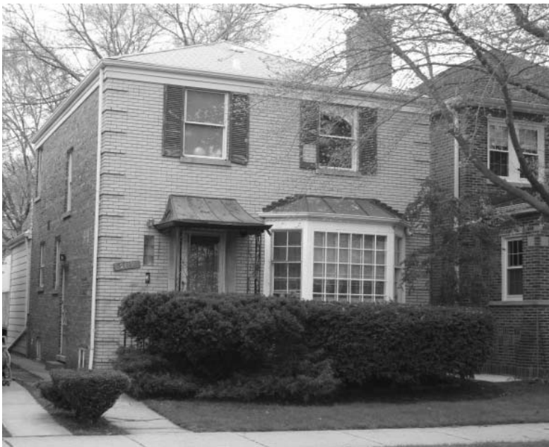
Current view of the Bell House, 2819 Sherwin
